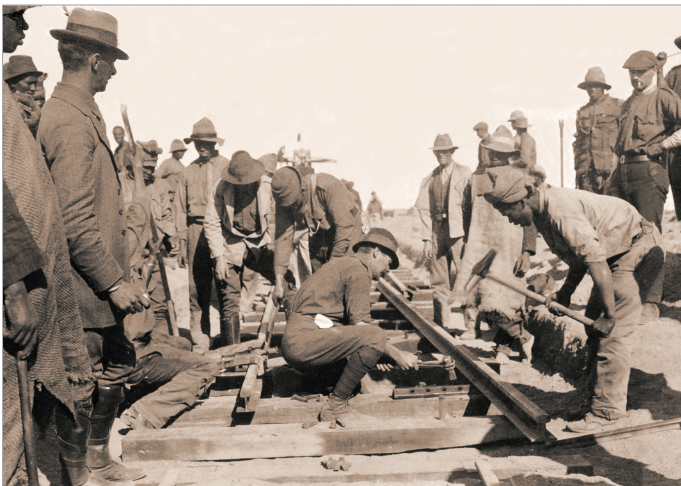
Figure 3: The last rail being laid before Kalkfontein; note the ends of the German rail at the bottom edge of the photograph (Transnet Heritage Library photograph GSWA020)
