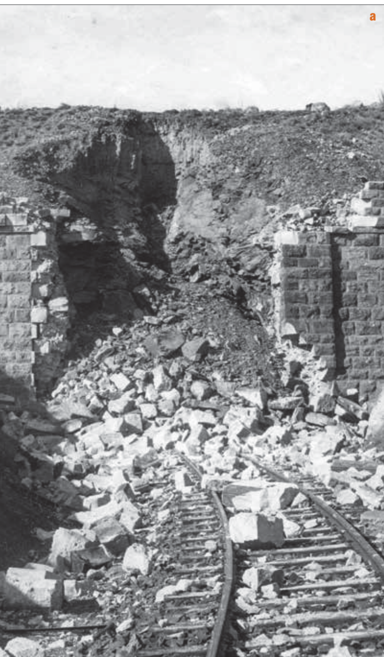
Figure 9: The damage inflicted on the Langsnek Tunnel during SA War 2: (a) the northern portal, with the shaft dug for the explosives in the background, and (b) the southern portal, which suffered less damage (Transnet Heritage Library, P3232)
