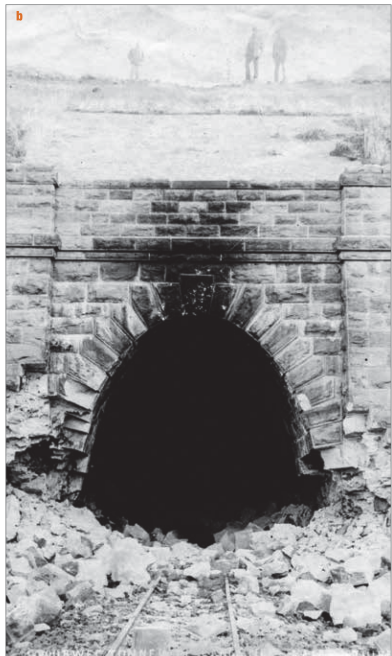
Figure 9: The damage inflicted on the Langsnek Tunnel during SA War 2: (a) the northern portal, with the shaft dug for the explosives in the background, and (b) the southern portal, which suffered less damage (Transnet Heritage Library, P3232)
