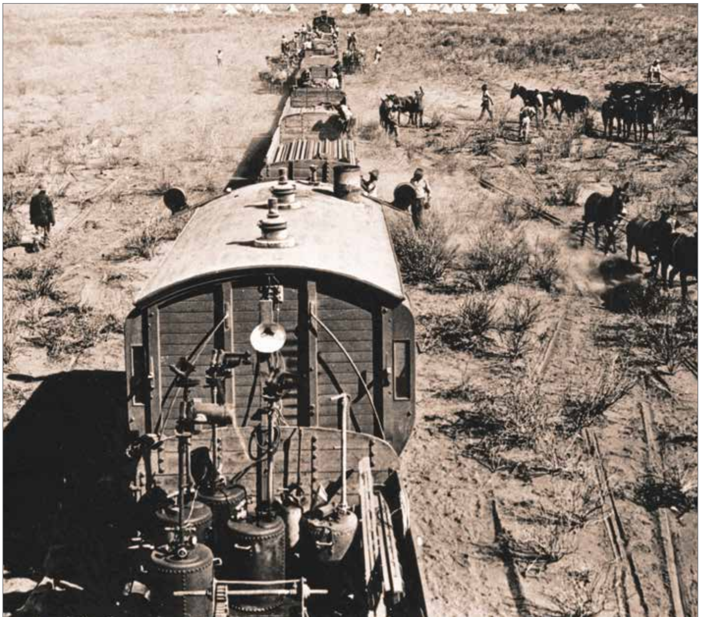
Figure 5: A material train being unloaded after being pushed up to the railhead by the locomotive in the background, with the tent camp for construction workers in the distance (Transnet Heritage Library photograph 18631)
