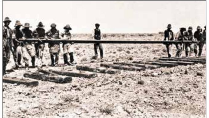
Figure 9: Rails were drawn to their approximate position by mules and chains before being placed by hand (Transnet Heritage Library photograph 18622A)
