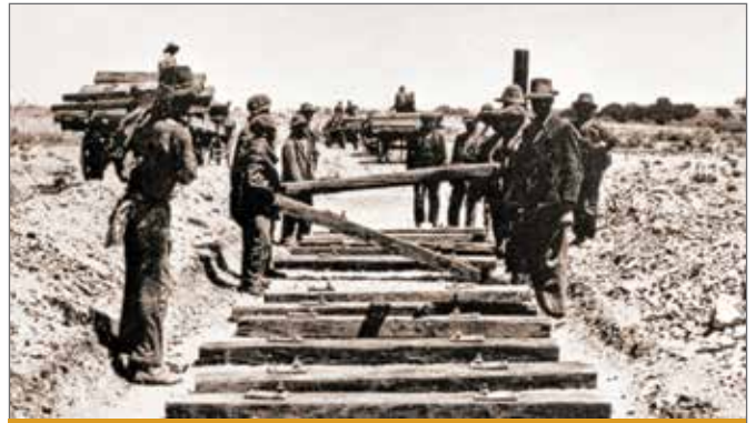
Figure 8: Sleepers were transported by wagon and placed by hand (Transnet Heritage Library photograph 18621)
