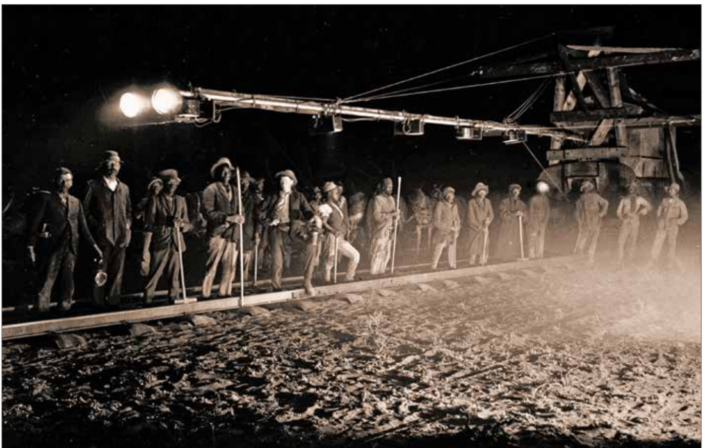
Figure 12: The lighting truck allowed working around the clock (Transnet Heritage Library photograph 18561)
