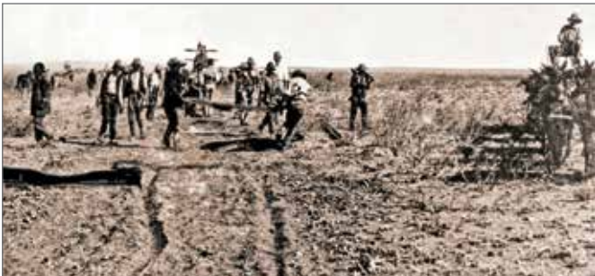
Figure 7: The track preparation on level ground was rudimentary with no compaction (Transnet Heritage Library photograph 18618)
